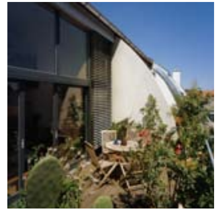
The roof-level apartments open up to the south into large terraces cut into the roof cladding.
